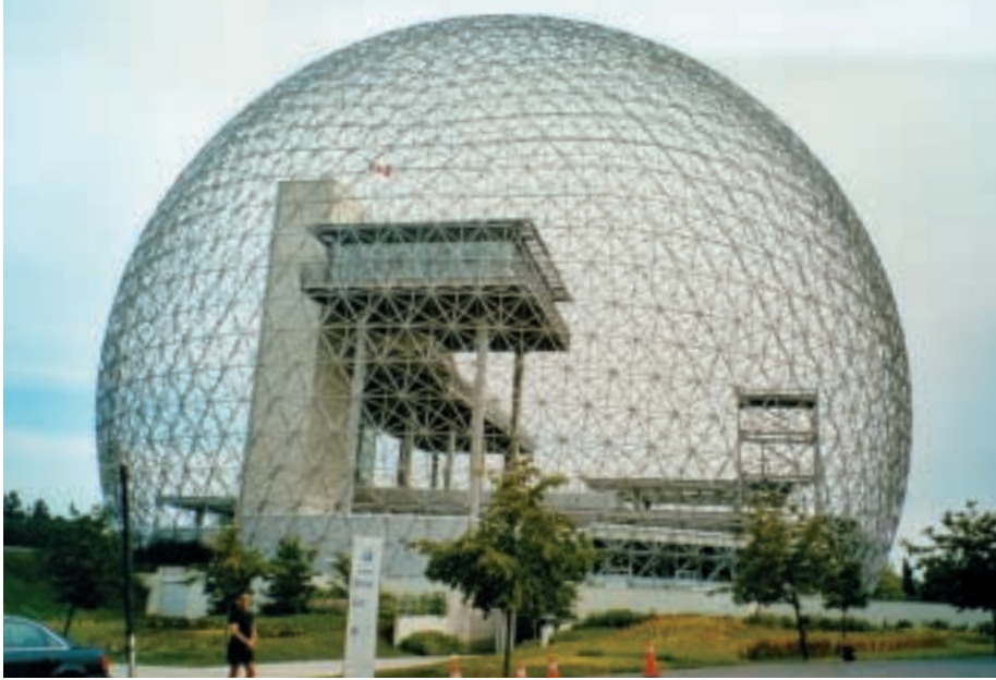
Fig. 1: Geodesic dome, 76 m in diameter, erected as the American pavilion for the 1967 World Fair in Montreal
